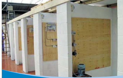
The new electrical bays in our training centre
